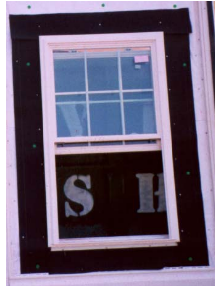
Figure 3 Flashing Detail
