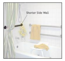
no more than 9" from the edge of the outside tub wall, with the bottom of the grab bar approximately 32" to 36" above the floor. A textured finish is recommended for a vertical grab bar as the hand may have a tendency to slip while wet.
