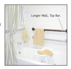
**Longer Wall, Lower Bar.** One 24" - 48" wide grab bar, installed 9" - 11" above the bathtub rim. This location offers a handgrip for pulling yourself up from the bathtub floor, transferring from or into a wheelchair, and getting up from a seated to a standing position when using a bath chair.
