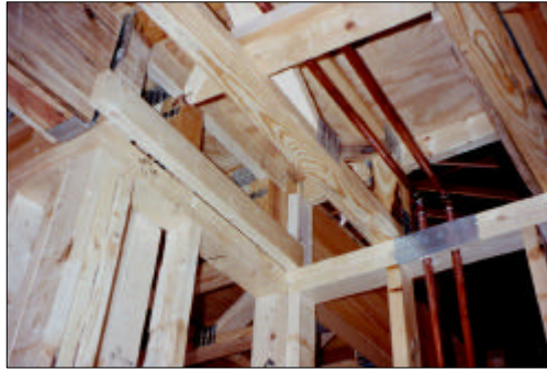
Holes in Plates
