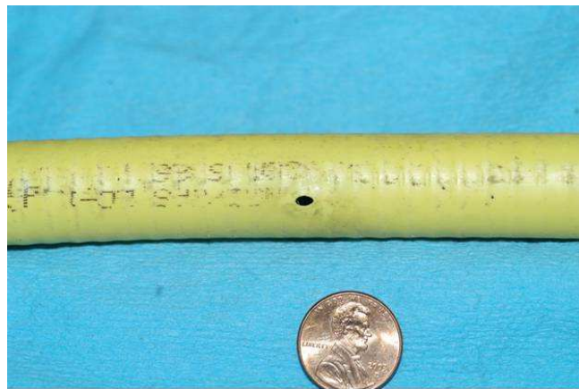
Figure 7: Photo of perforated CSST without pyrolysis
