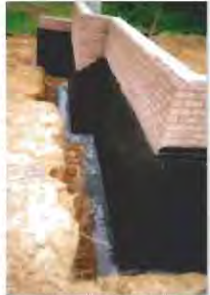
Foundation Wall using Amerdrain Sheet Drain
