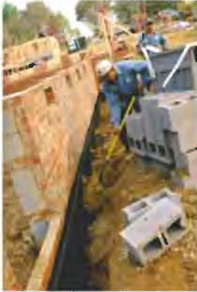
Foundation Footing using Akwadrain™ Strip Drain
