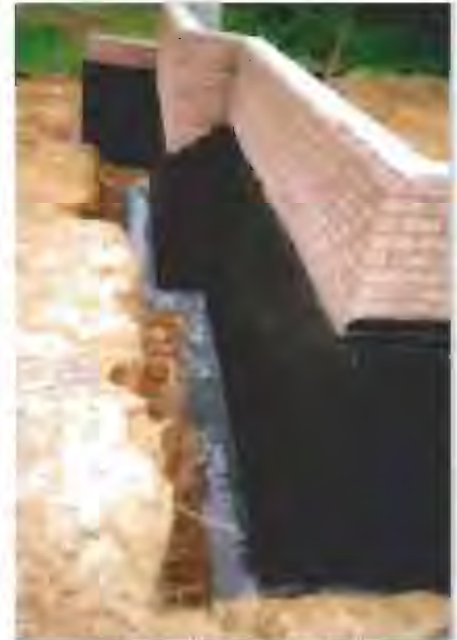
Foundation Wall using Amerdrain Sheet Drain
